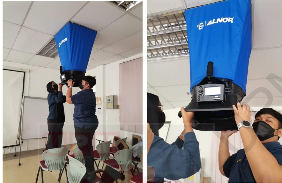
Figure 3.8. The measurement of air velocity from an air inlet of tutorial room using Alnor TSI Balometer Capture Hood EBT731
