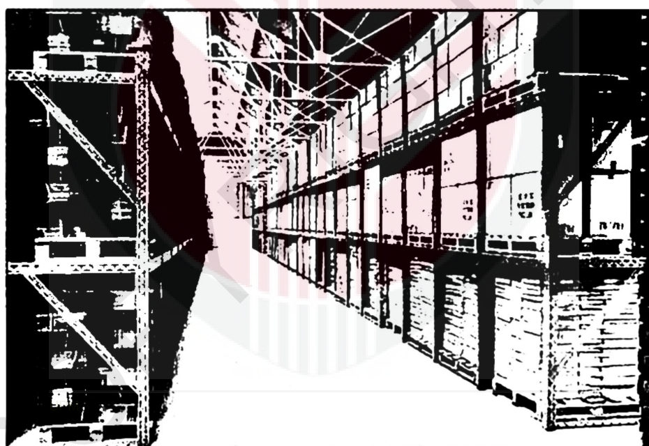
Figure 4.14: Pallet racking in chiller storage room.
