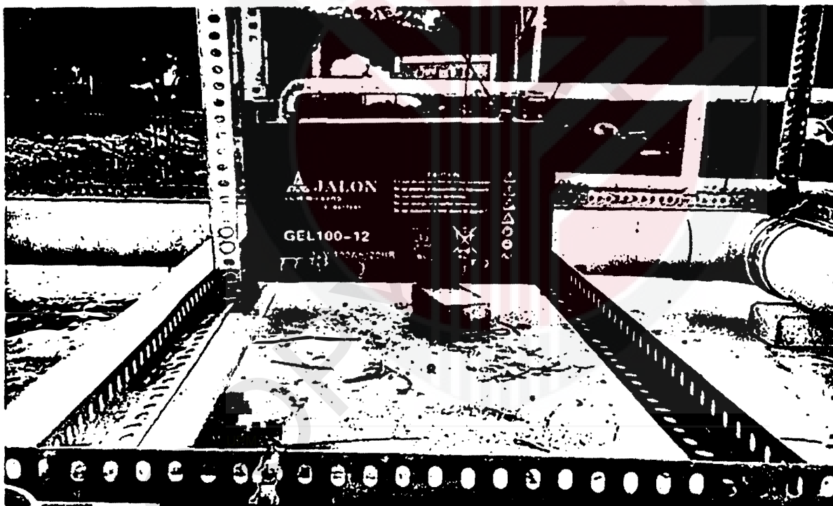
Figure 4.8: Additional compartment for battery placement
