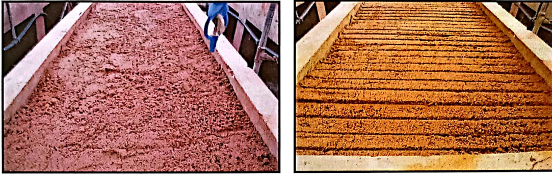
Figure 3.1: Sand Bed Preparation
