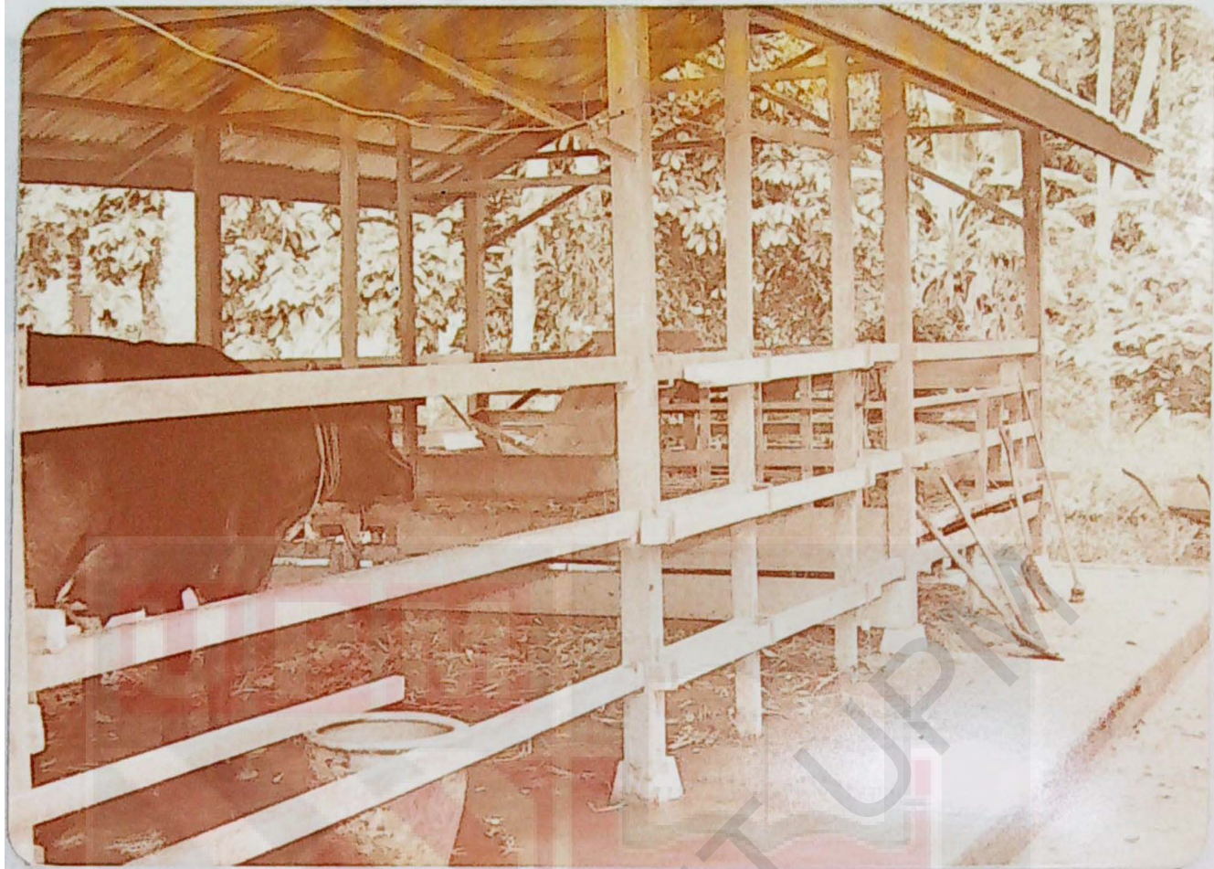
A well constructed shed belonging to a bachelor Encik Md. Ior Kosai in Muar. Notice the cement floor, zinc roof, sawn wood and separate and raised calf-per. Cleaning equipment and water container can also be seen.
