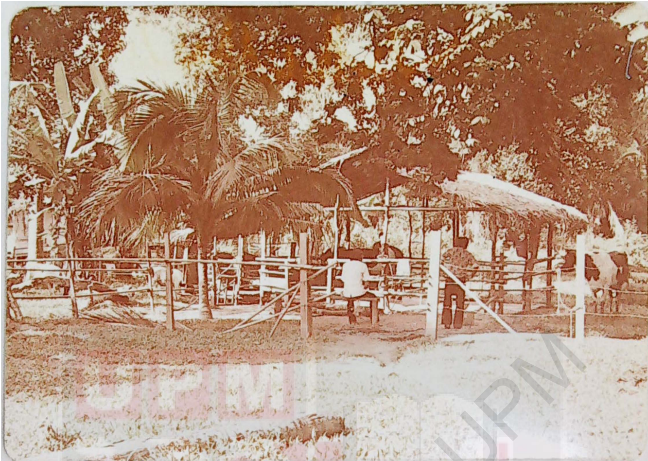
A Kampung Malay cattle shed in the backyard. Notice the thatched roof and the jungle wood use for construction. The floor is cemented and the calf-pen is partitioned on the left. The fruit tree canopy provides shade for holding the cattle before the afternoon grazing.
