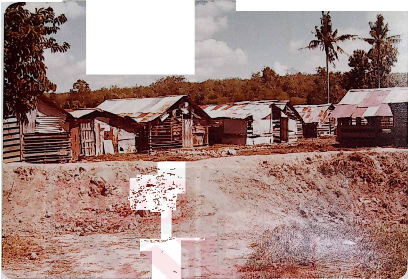
Cattle shed in estates. Notice the poor arrangement of the sheds, the low roofs and the scrap materials used for construction.
