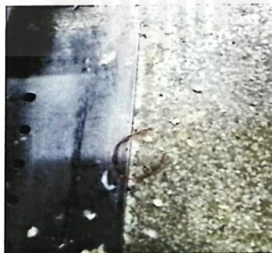
Figure 4.4 1: accumulation of soils at floor-drain interface
