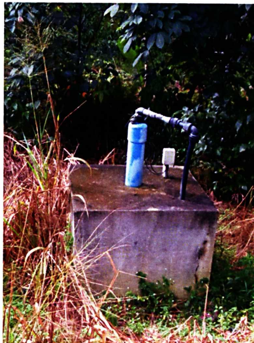
Tube well that had been sealed and closed
