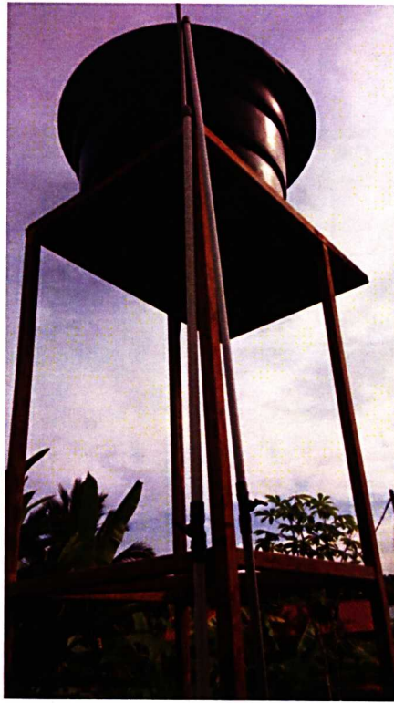
Water tank for groundwater storage at respondents' houses
