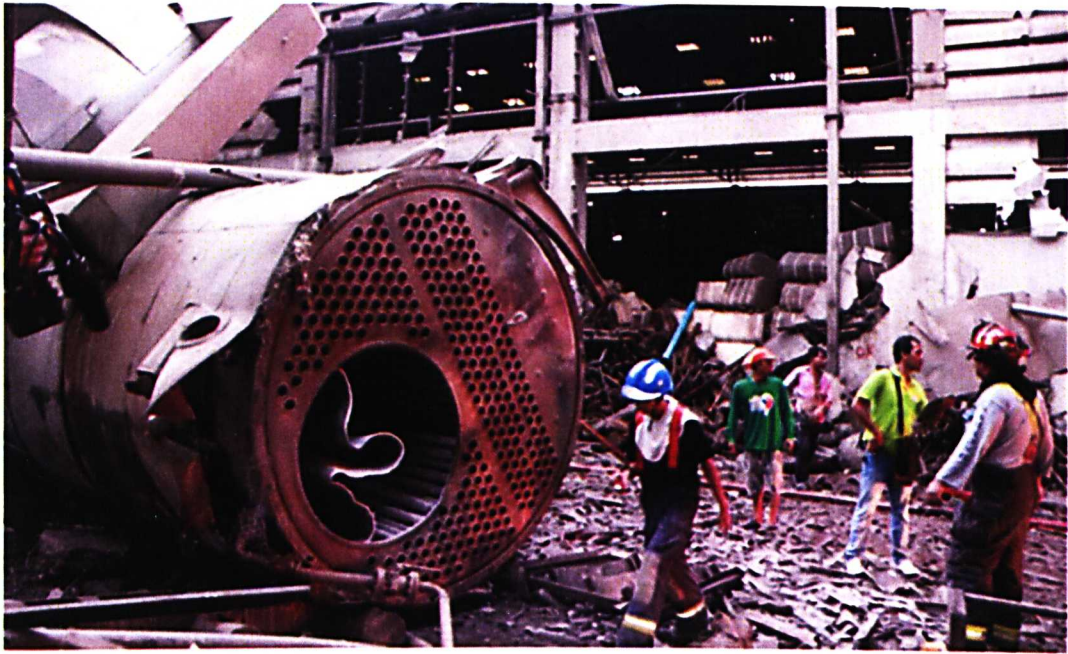
Figure 2.5: Steam Boiler Explosion in Thailand, 2014 (Source: http://www.thewbia.com/WP/boiler-accidents/ )
